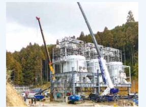
Installation of dry distillation gasification combustion plant systems
